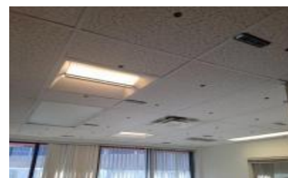
In an effort to study the effects of lighting on human health and diseases, the Smart Lighting Engineering Research Center (ERC) at Rensselaer Polytechnic Institute (RPI) recently installed a novel hospital inpatient lighting test bed for the study of automated lighting at the University of New Mexico Health Center
